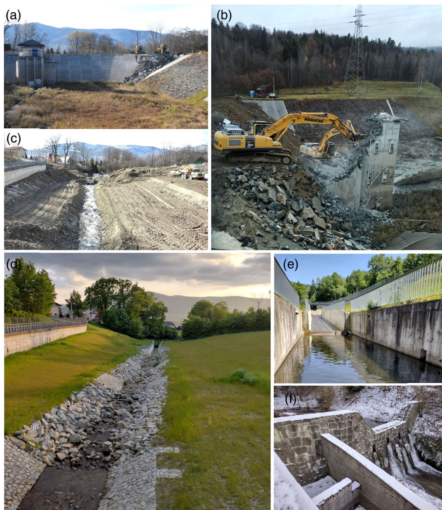
PHOTO 1 Course of Wilkówka dam removal and stream condition after removal: (a) decommissioning works begin, November 2021; (b) demolishing the tower chute, November 2021; (c) earthworks on the former dam and reservoir in February 2022; (d) area after completion of demolition works, June 2023; (e) barrier in riverbed (remnant of frontal dam), June 2023 and (f) debris dam in the former reservoir backwater, February 2023 (phot. M. Habel). [Colour figure can be viewed at wileyonlinelibrary.com ]
